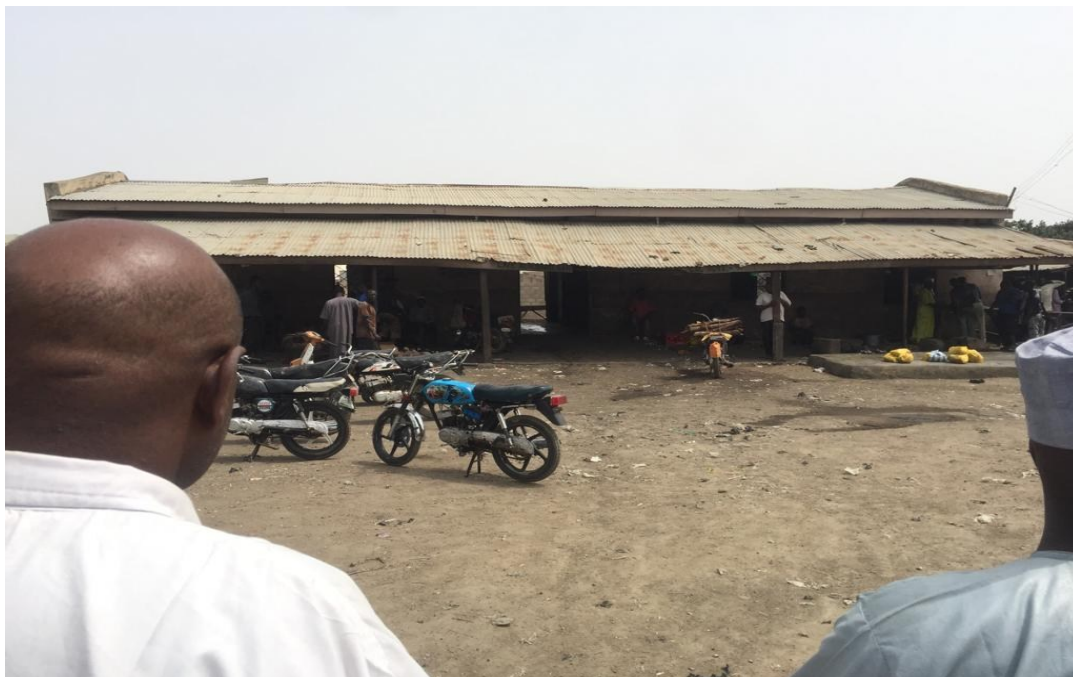
Plate 1: The picture shown Tarauni Slaughterhouse in Tarauni local government Kano state which currently not architecturally well-defined
