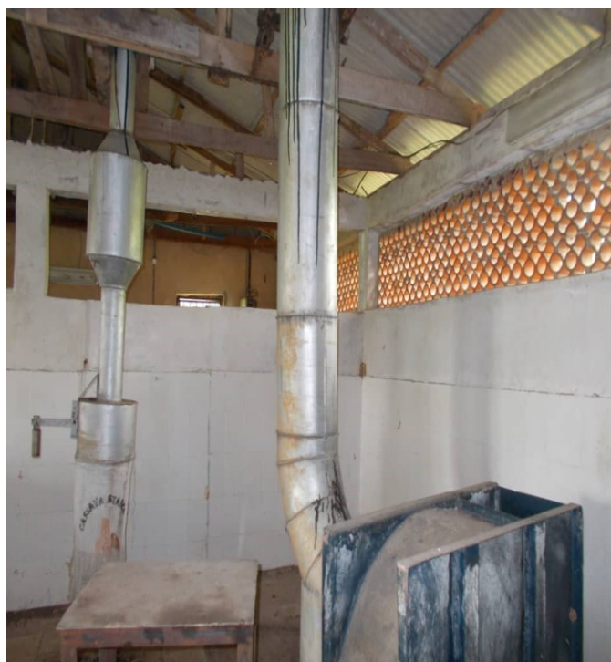
Plate 2: The Flash Dryer process showing Heat Exchanger
