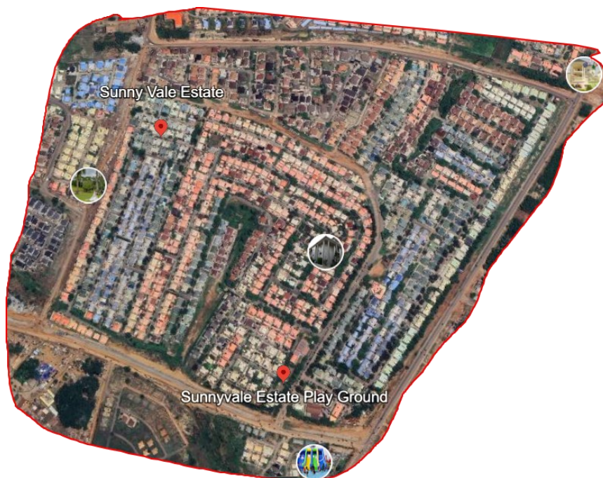
Figure 1: Aerial View of Sunnyvale Estate Mass Housing Development Source: https://earth.google.com/ (Retrieved April, 2024)
