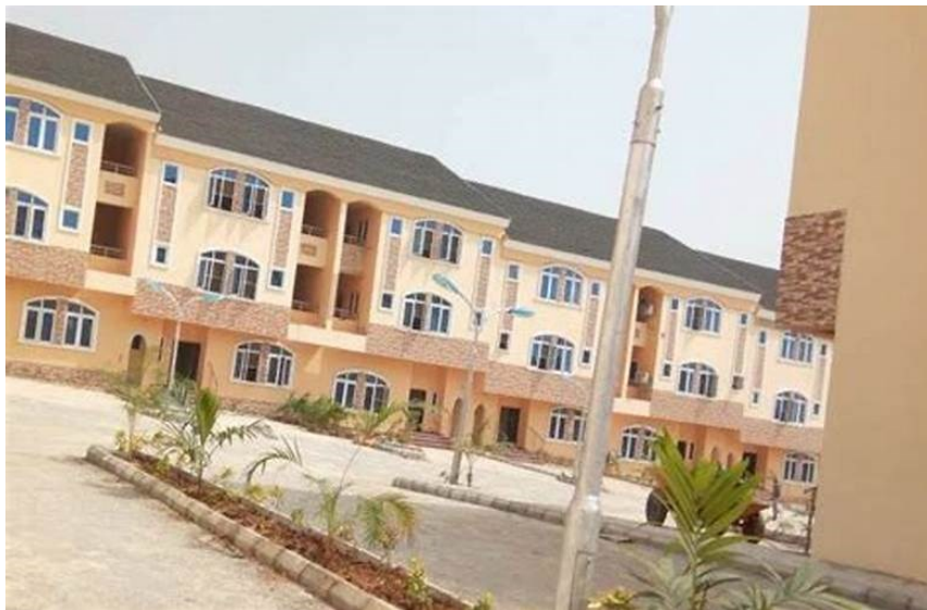
Figure 6: Life-Camp Condominium Mass Housing Development
